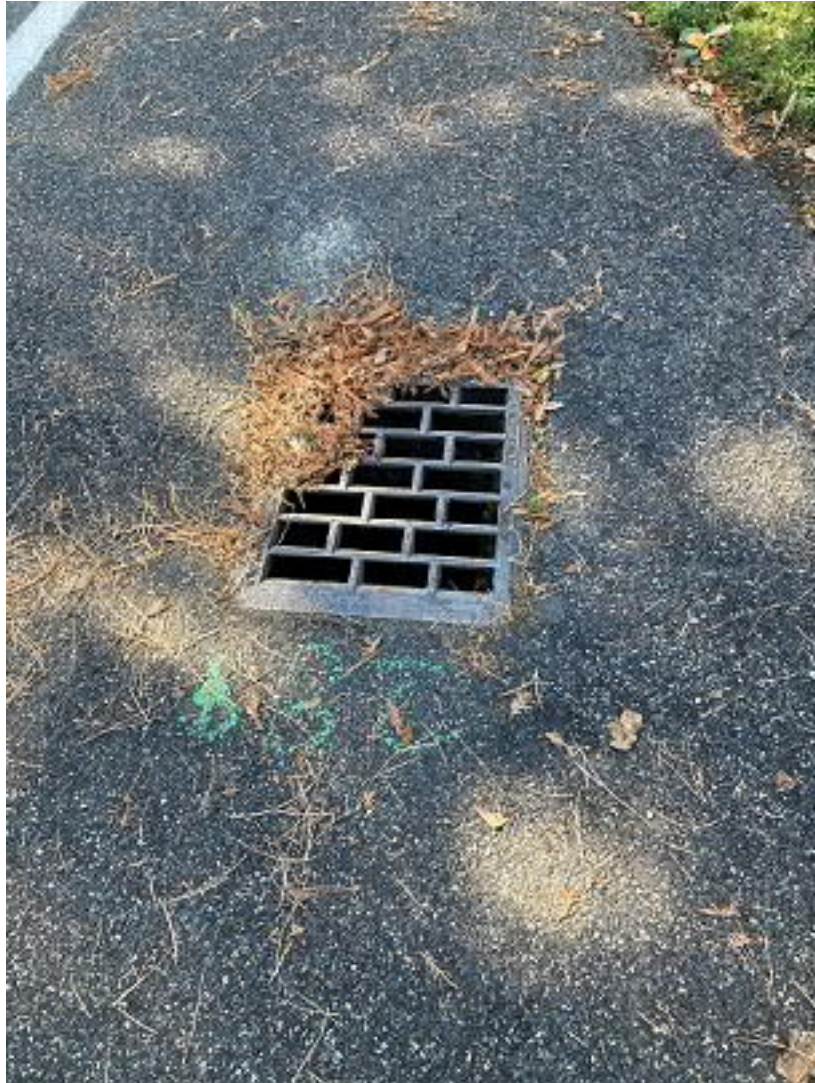
Picture 2: westernmost corner of Mercerwood Drive and SE 43 rd Place Catch basin across 43 rd Place SE from the first one.
